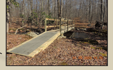
BRIDGE CROSSING GRISCOM RUN
